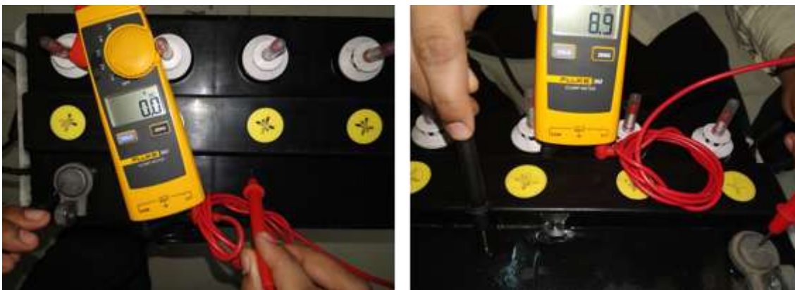
Figure 54 Measuring of leakage voltage on clean and unclean battery soiled with electrolyte
