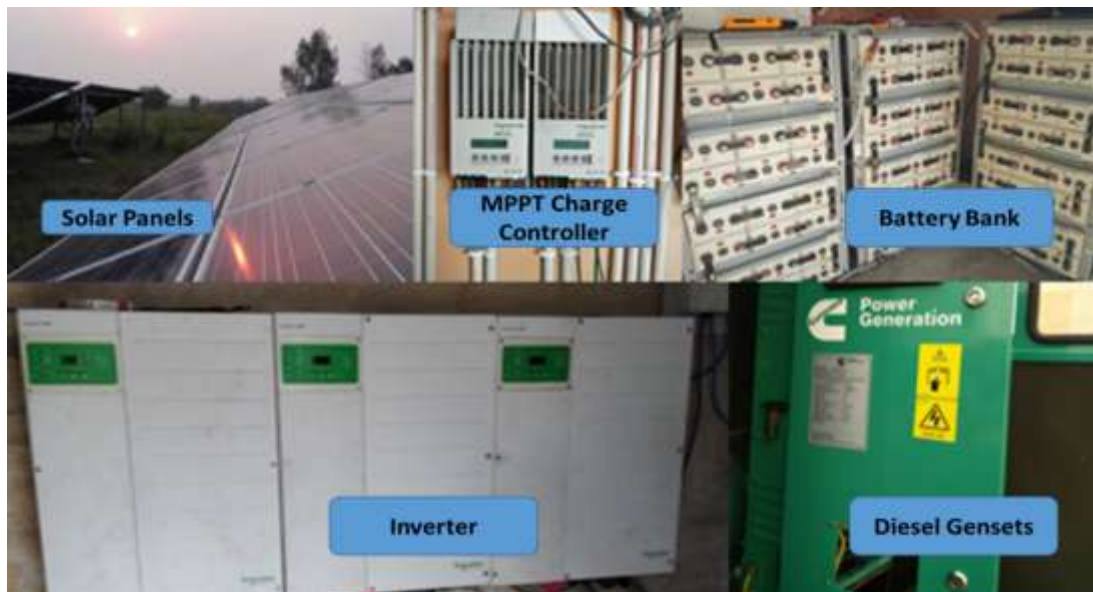
Figure 3 Image collage of an off-grid solar PV microgrid (source: CES)
