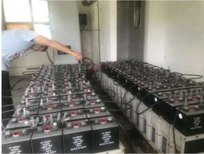
Figure 65 Battery output data in kWh for site 4 before and after equalization (Source: CES)
