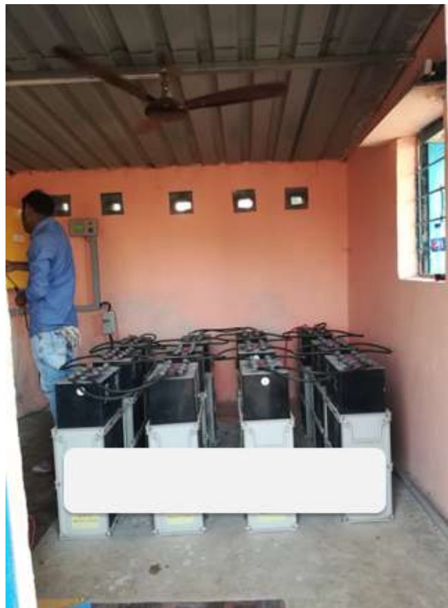
Figure 60 Flooded tubular battery bank at site 1 (source: CES)
