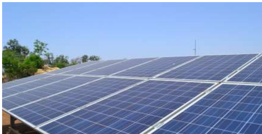
Figure 6 Solar PV panel array at a rural microgrid (source: CES)
