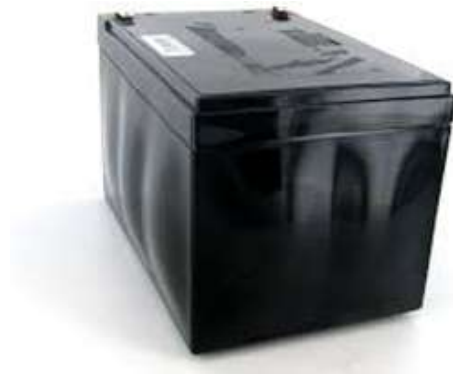
Figure 33 Bulging of Battery with Over Charging
