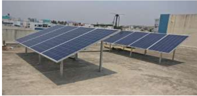
Figure 1 2.4 kWp solar PV plant at the lab (source: CES)
