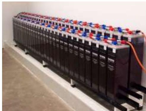
Figure 21 Photograph of a battery bank comprising of 2 V flooded tubular cells
