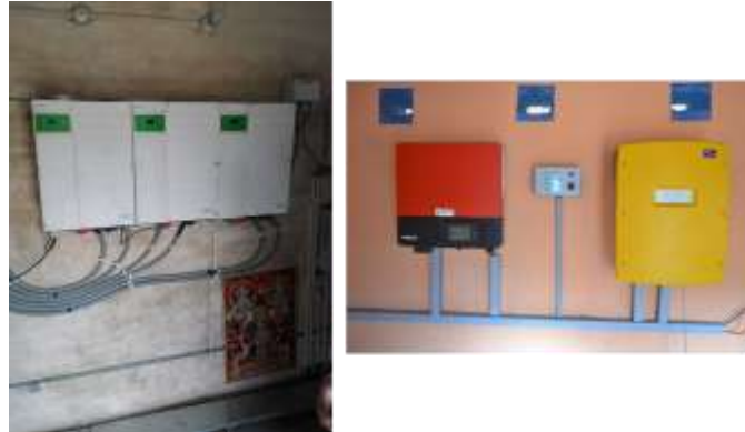
Figure 12 Solar PV Inverters and Battery Inverters at DC coupled (L) and AC coupled (R) Microgrids (Source: CES)
