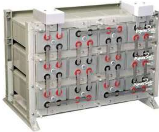
Figure 25 Photograph of a 24 V battery bank comprising of 2 V AGM cells (source: CES)
