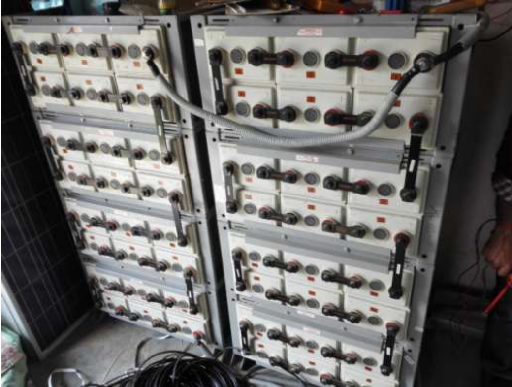
Figure 63 AGM battery bank at site 2 (source: CES)
