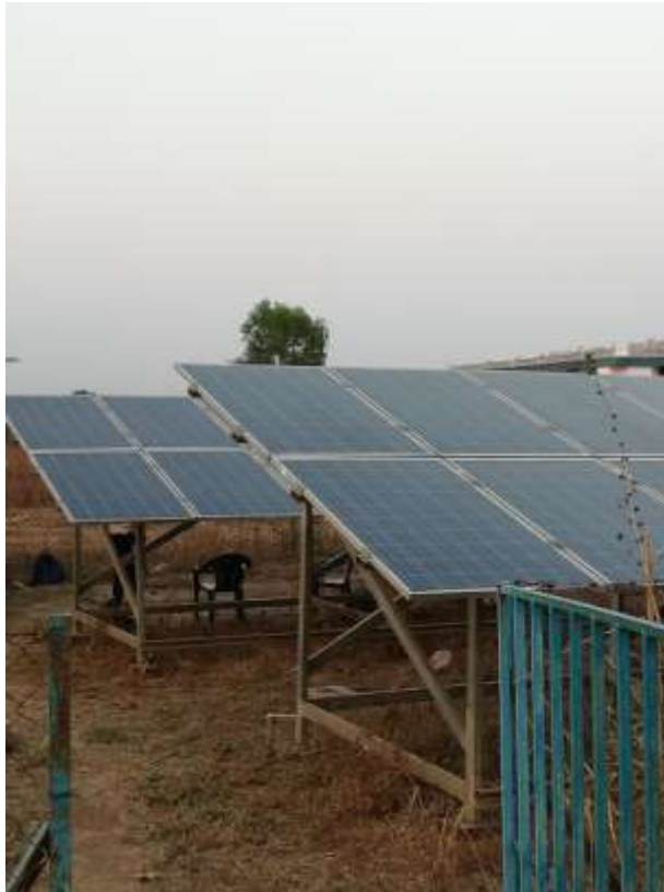
Figure 61 Solar panels at Site 1 (source: CES)
