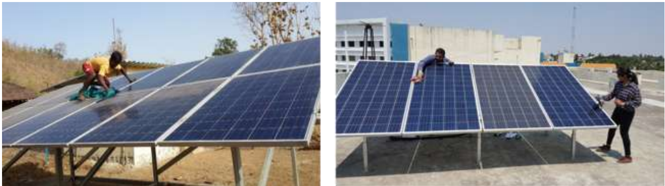
Figure 30 Cleaning of solar PV panel at a rural micro-grid and at solar rooftop PV plant (source: CES)
